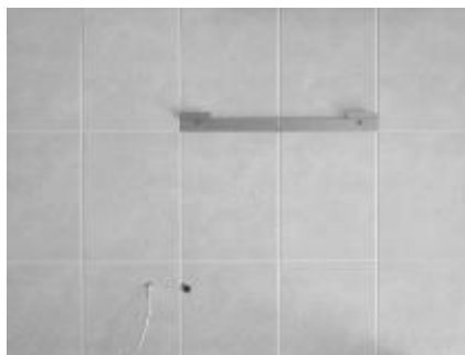
Preparation of electric power supply, condensate drain and console mounting
